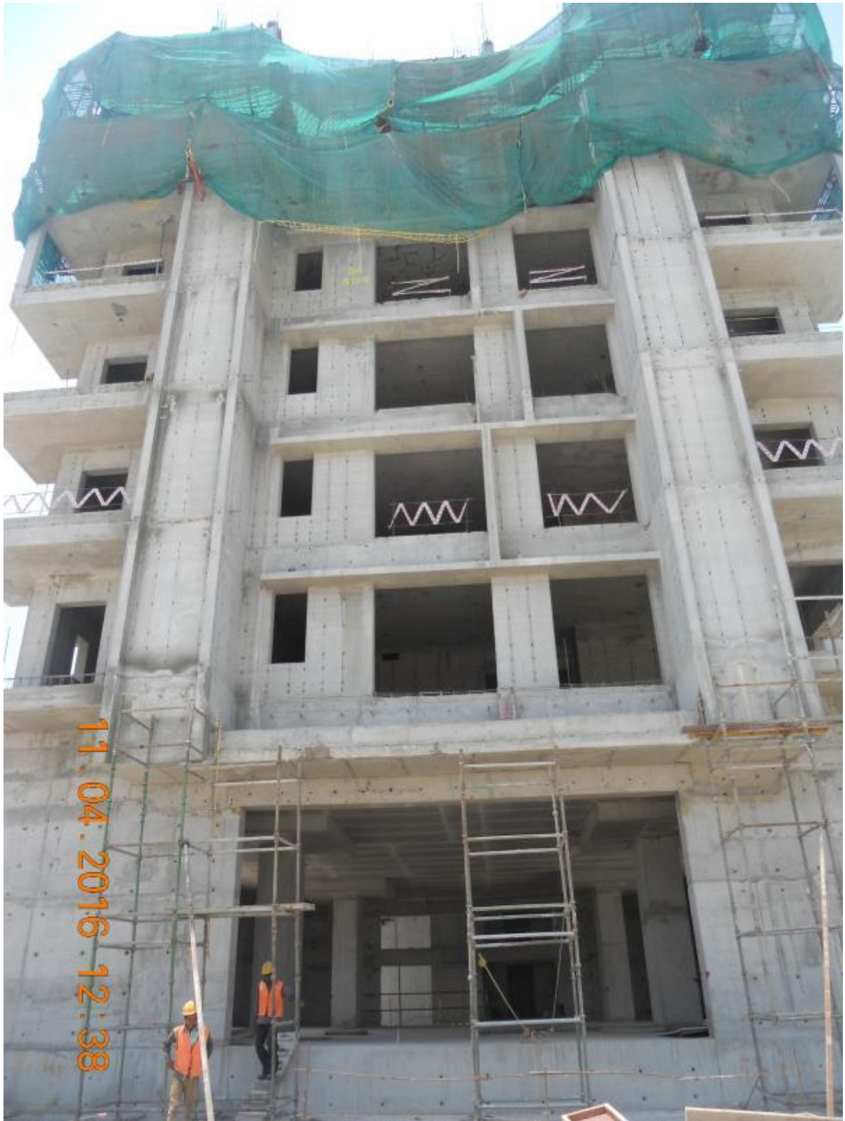
EAST VIEW OF BLOCK A
