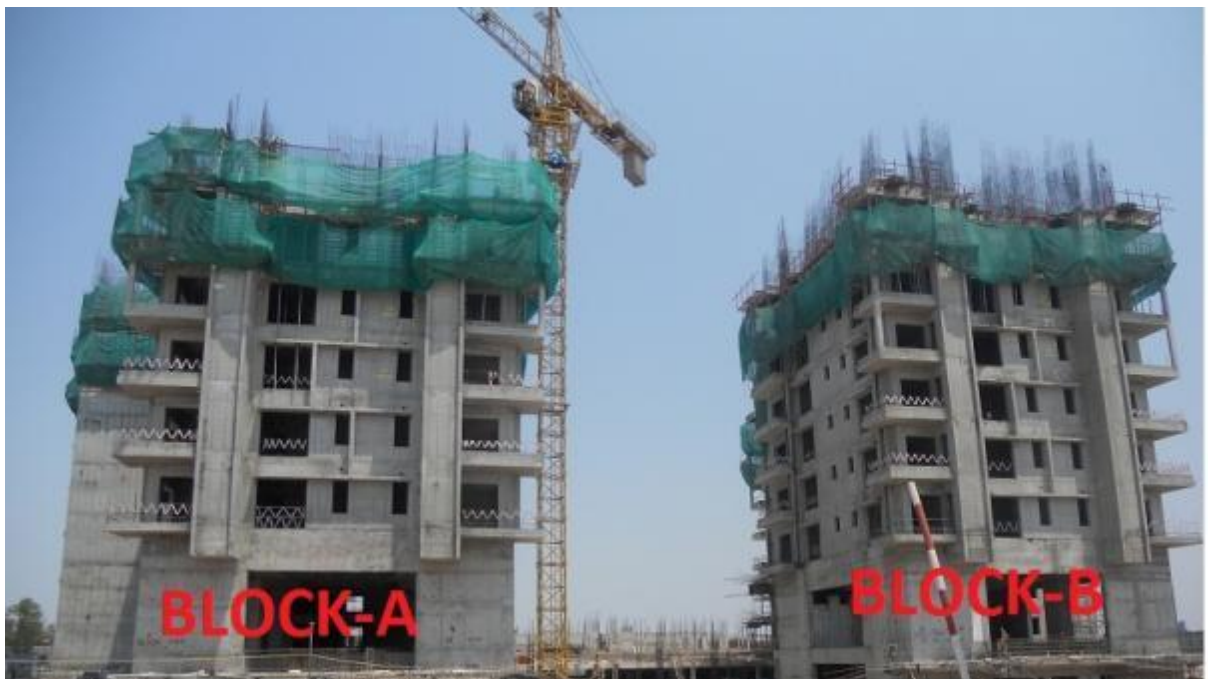
WEST VIEW OF BLOCK A & B
